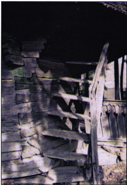
Joints in the sector of the access ladder to the attic and the porch ending, at the end of the pronaos - Fânațele Silvașului de Câmpie
