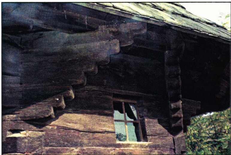
"Dovetail joints" at the apse apsis - the wooden church at Bungard
