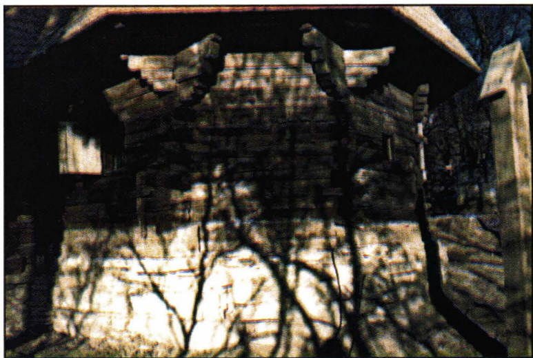
Dovetail joints - Runcu Salvei
